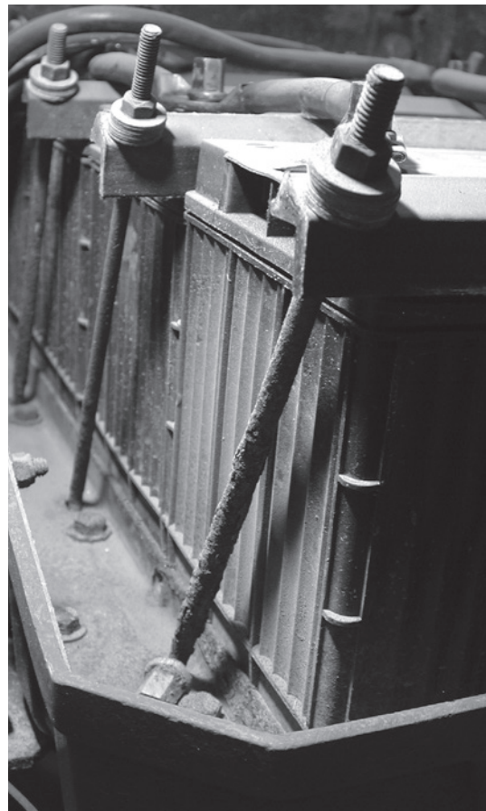
Make certain that battery hold-downs are tight enough to hold the batteries securely.
