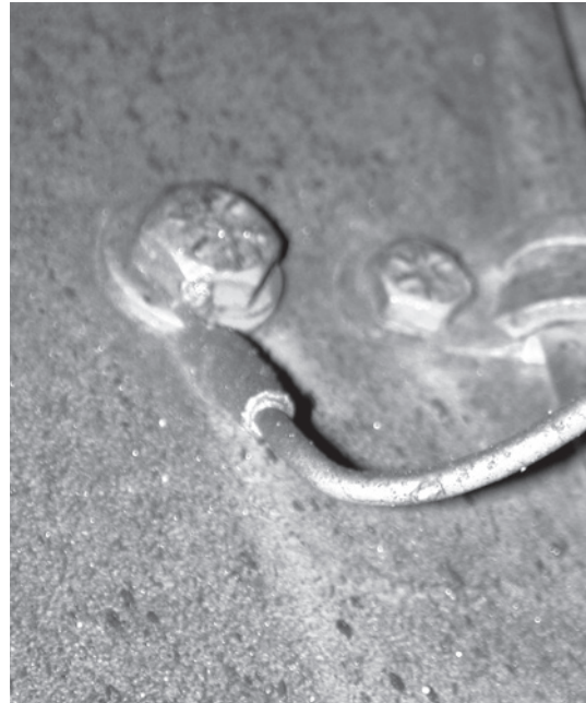
Since dirt and corrosion are ever-present enemies, care should be taken to make sure that a proper ground is securely made.
