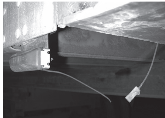
Too much stress on a wire may cause conductors to break, crimps to give way, and connections to pullout resulting in failure.
