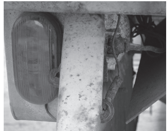
In most trailer applications, the connections from the lighting devices are open to the elements.
