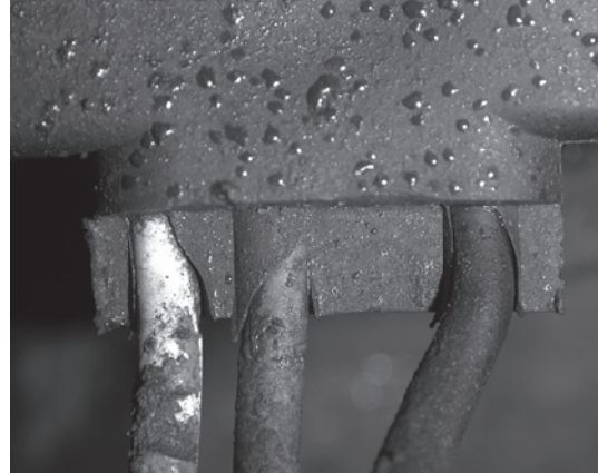
In some cases, sand and grit may work their way inside protective coverings and abrade the insulation of wires.
