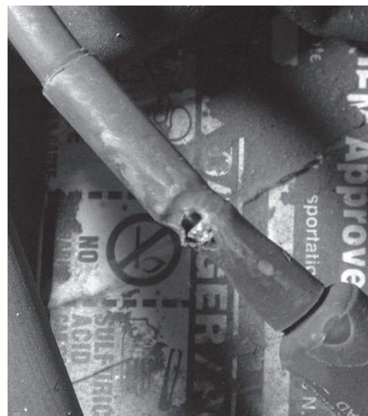
Visually inspect the battery cables for worn insulation that will expose the conductor to moisture and corrosion.
