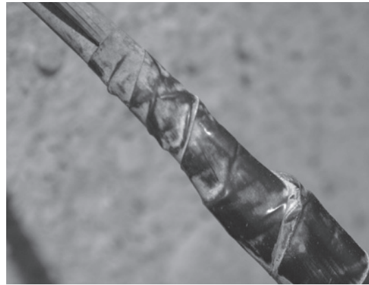
Do not use electrical tape alone to secure and seal connections.
